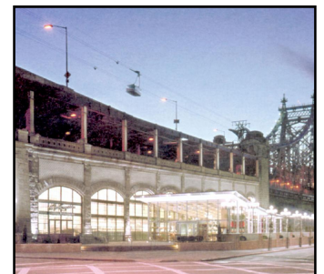
59th Bridge, New York City
