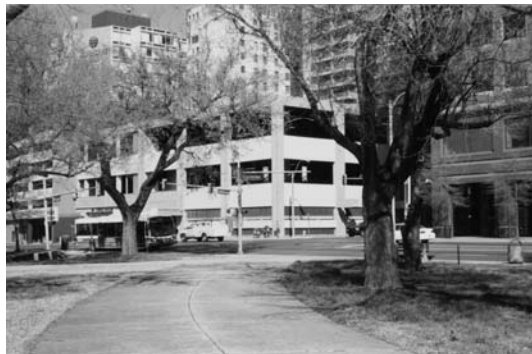
A large parking structure is located at the northeast corner of Front Street and Jefferson Avenue. Jefferson Avenue has been designated as the main link to the future Land Bridge from downtown.
